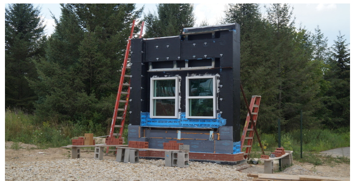
Materials testing mockup. To save on cost and time, smaller mockups of the envelope of a building will be produced to test various flashing, insulation materials, window installations and other variables to ensure proper function. Any issues are then resolved on a smaller scale prior to installation on an entire building. This particular mockup was rigorously tested for flashing installation, brick adherence and appearance, vapor barrier effectiveness and window sealant quality.
